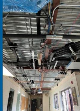
HVAC Piping insulation complete upper level 2011
